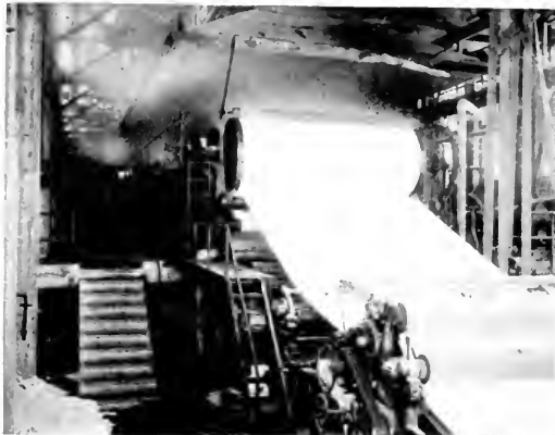
Dry End, Pulp Drying Machine.
